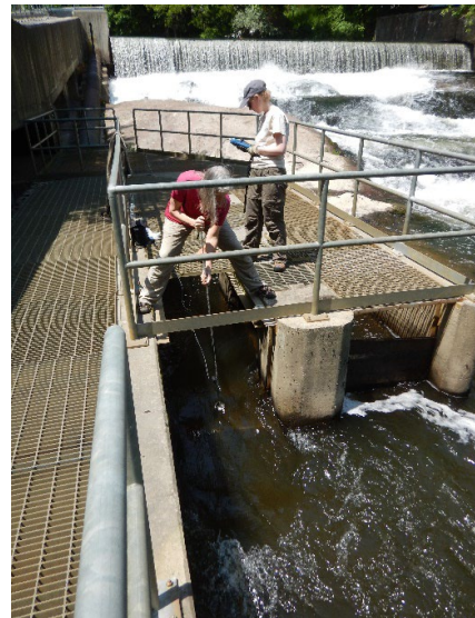
Image 1. FWS Fish Passage Engineer Jessica Pica and Melissa Grader (Hydropower Team) setting the proper entrance conditions at the Manhan River Fish Ladder this week.
